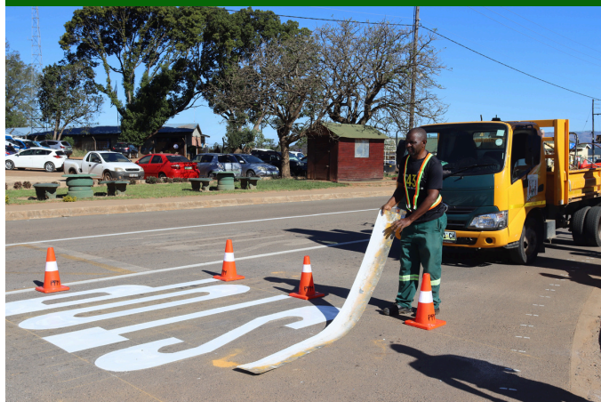
Maintenance of MRI Road
